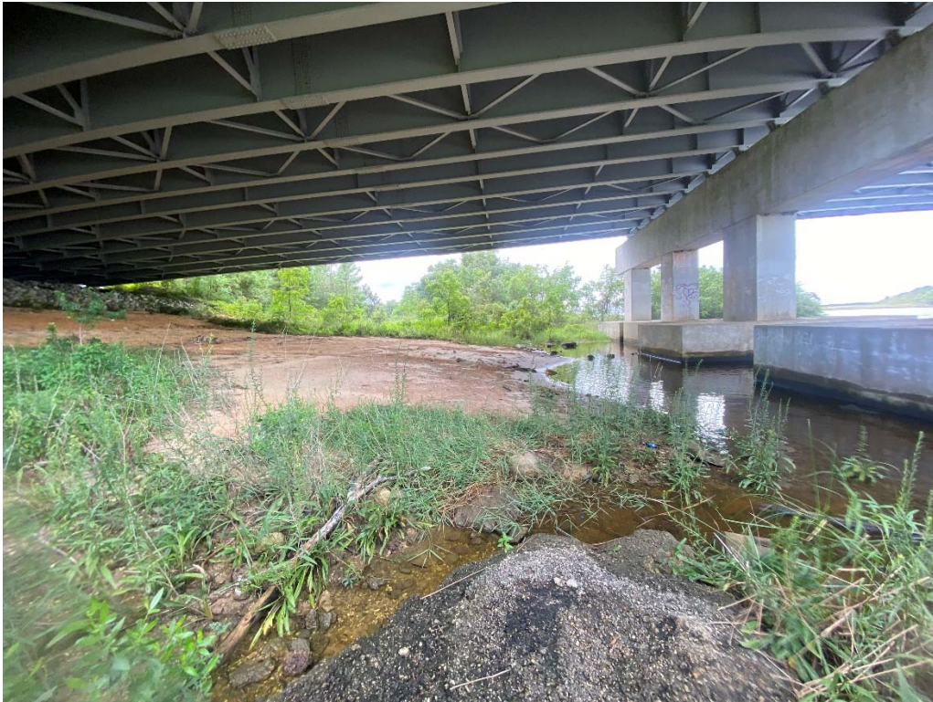
Figure 5-4: Akoko Street Extension – Existing I-10 Bridge (Looking South)
