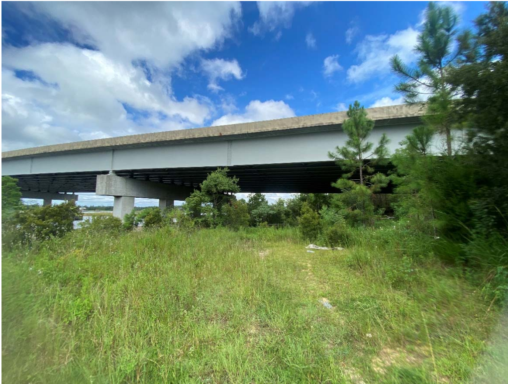
Figure 5-3: Akoko Street Extension – Existing I-10 Bridge (Looking North)
