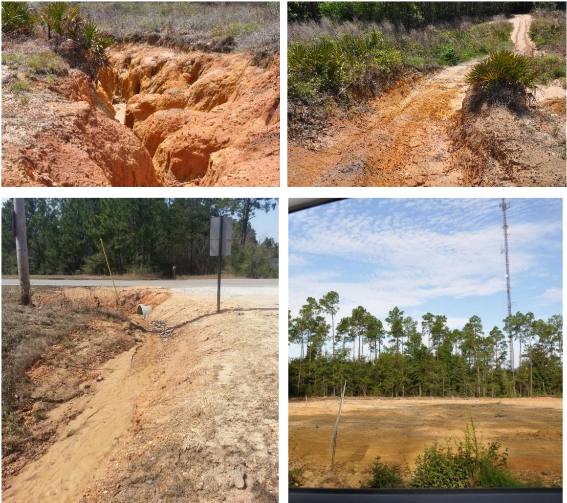
Figure 12: Erosion in Rotten Bayou Watershed
