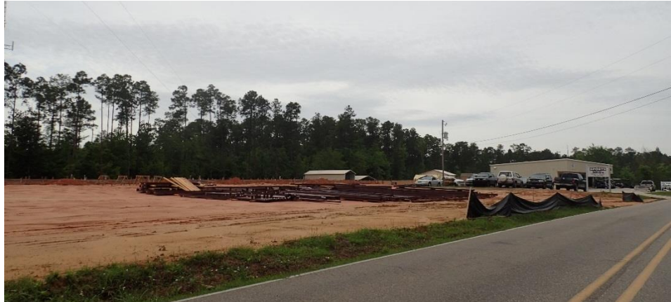
Figure 15: Active Construction Site in Rotten Bayou Watershed
